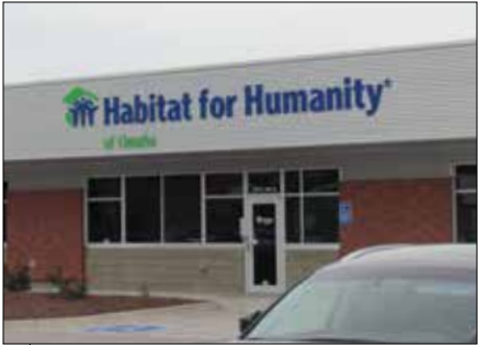
In 2000, the Habitat Omaha office and warehouse moved to a much newer office and warehouse combination building. The new building, at 1701 N. 24th Street, thrilled the construction staff and office staff with about three times as much space. No one used a card table for a desk, most people worked in cubes and a few people enjoyed offices. The copier, well, several copiers now, had their own corners. Each Habitat truck had its own parking space with easy in and out access. Eventually we outgrew this office space, too.
