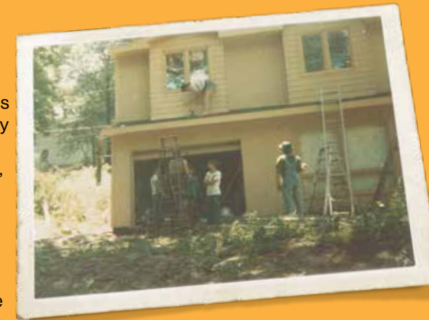
Work being done on the first Habitat Omaha home build, located at 3711 Spencer Street
