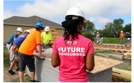
Trained staff and crew leaders supervise home construction, with volunteers and future homeowners contributing most of the labor.
