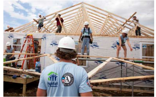
Trained staff and crew leaders supervise home construction, with volunteers and future homeowners contributing most of the labor.
